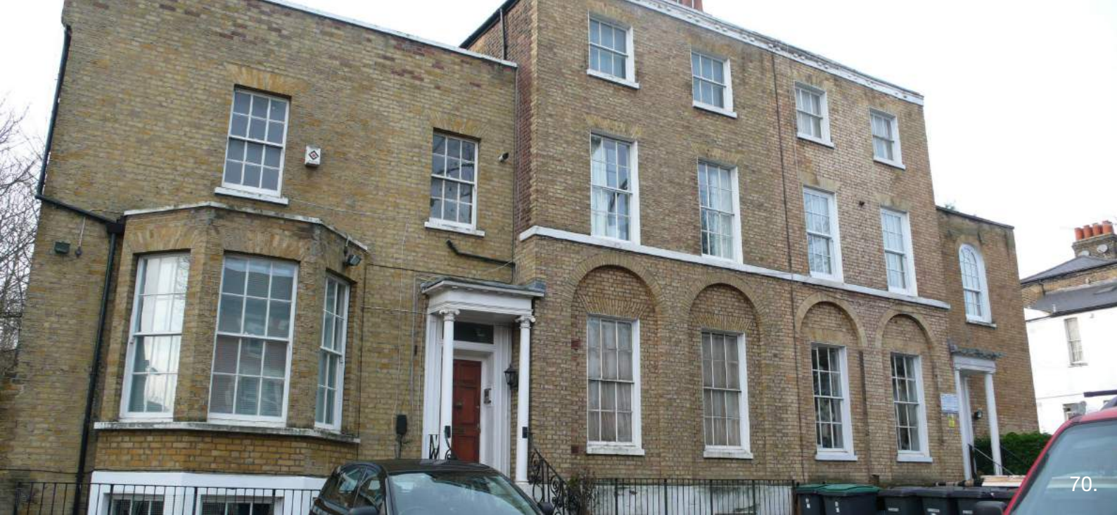
Picture 75. 11 and 12 Bruce Grove - Grade II listed
