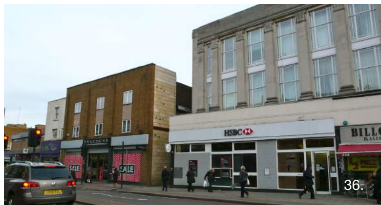
Picture 34. 482-488 High Road, showing the oversized fascia at No.488
